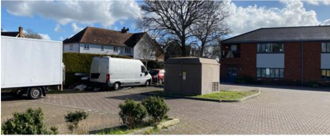
Carriers Way electrical substation
