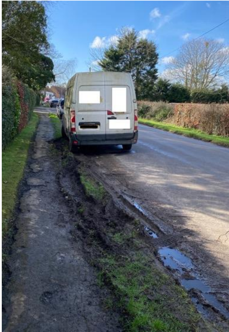
Damage to Verges on Waldron Road
