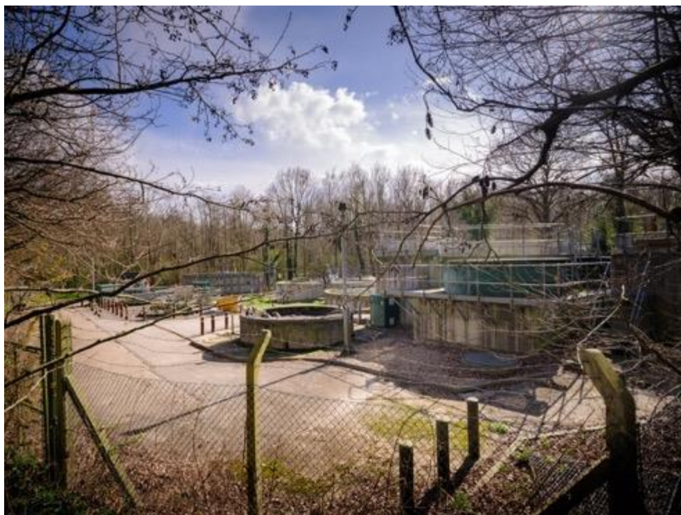
East Hoathly Sewage Treatment Plant
