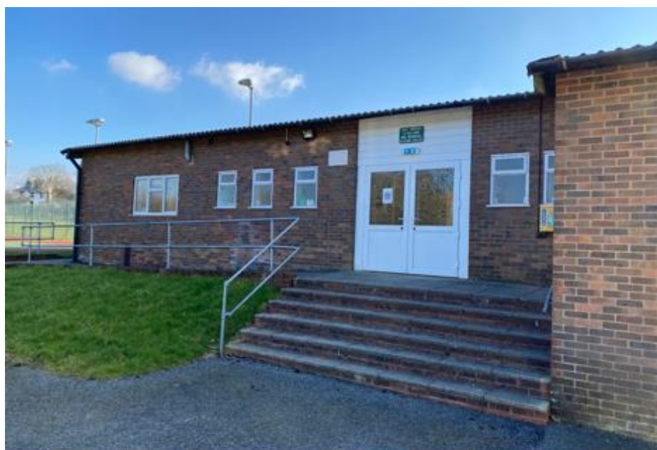
View of Pavilion from Car Park
