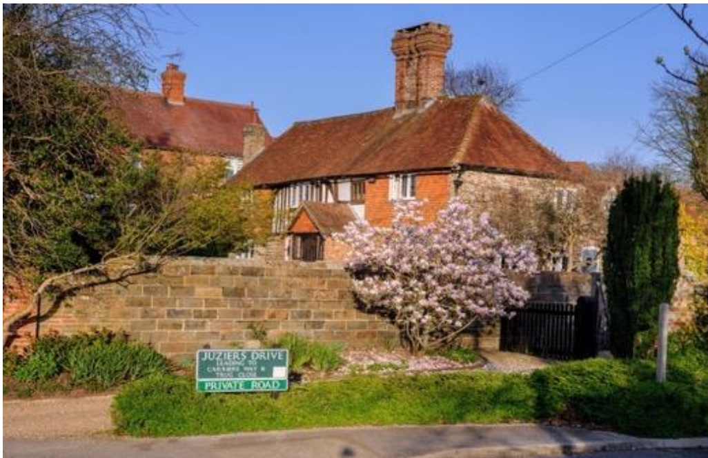
Sellens Cottage - Probable 15th Century Medieval Hall with floor and chimney added in 16th Century.
