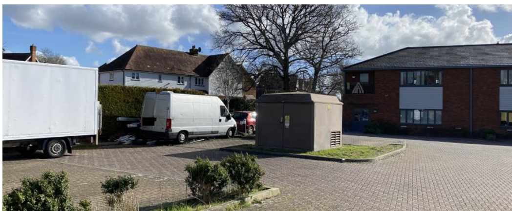
Carriers Way electrical substation
