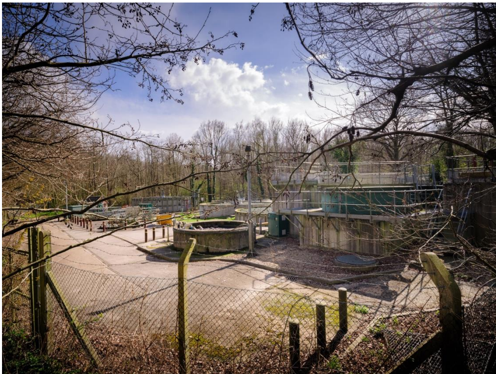
East Hoathly Sewage Treatment Plant
