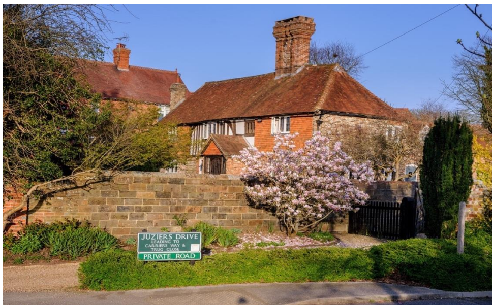
Sellens Cottage - Probable 15th Century Medieval Hall with floor and chimney added in 16th Century.
